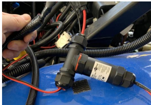
Figure 12: Better protection for cabling, March 2023
